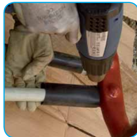
Fixing the heat-shrink sheath between cable and header.
