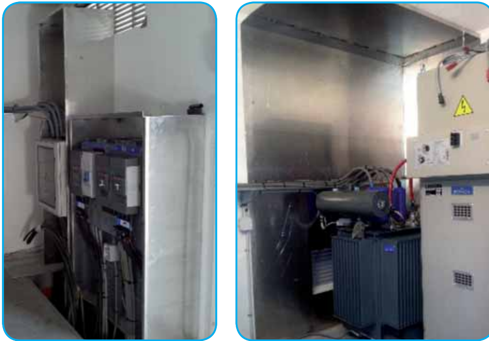
Fig. 18 - Shielding element installation
