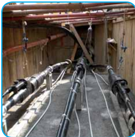
Start of the shielding cable positioning stage.
