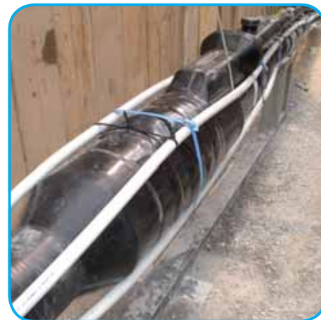
Shielding cables near the HV cable joint.
