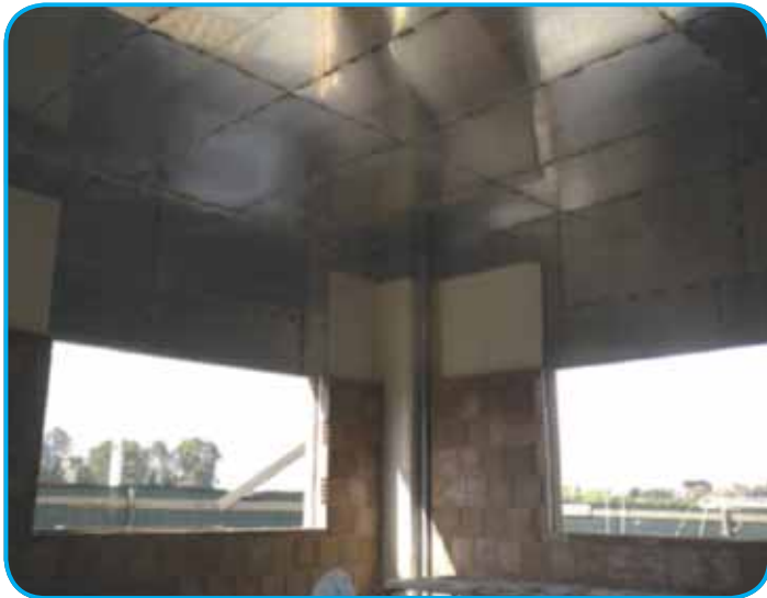
Fig. 11 - Installation of the shielding
