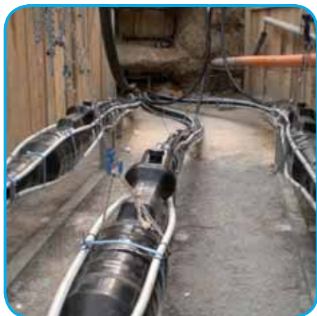
Shielding cables installed on all HV cables.
