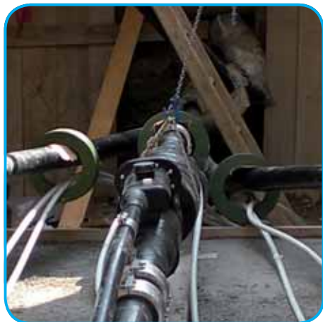
Toroids on the three phases.
