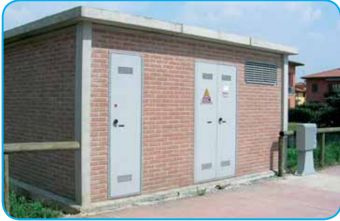
Fig. 16 - Secondary transformer substation
